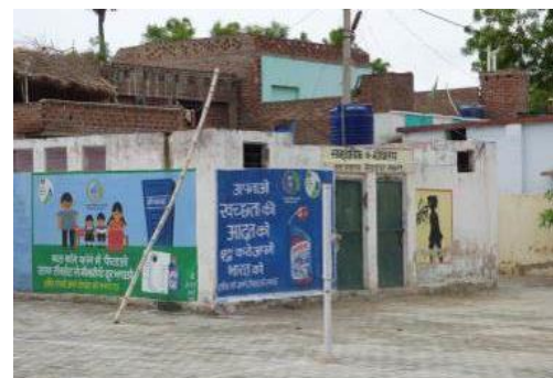
The toilets of the Panchayati Bhawan in Sayyedpur Shekhri, Kannauj
